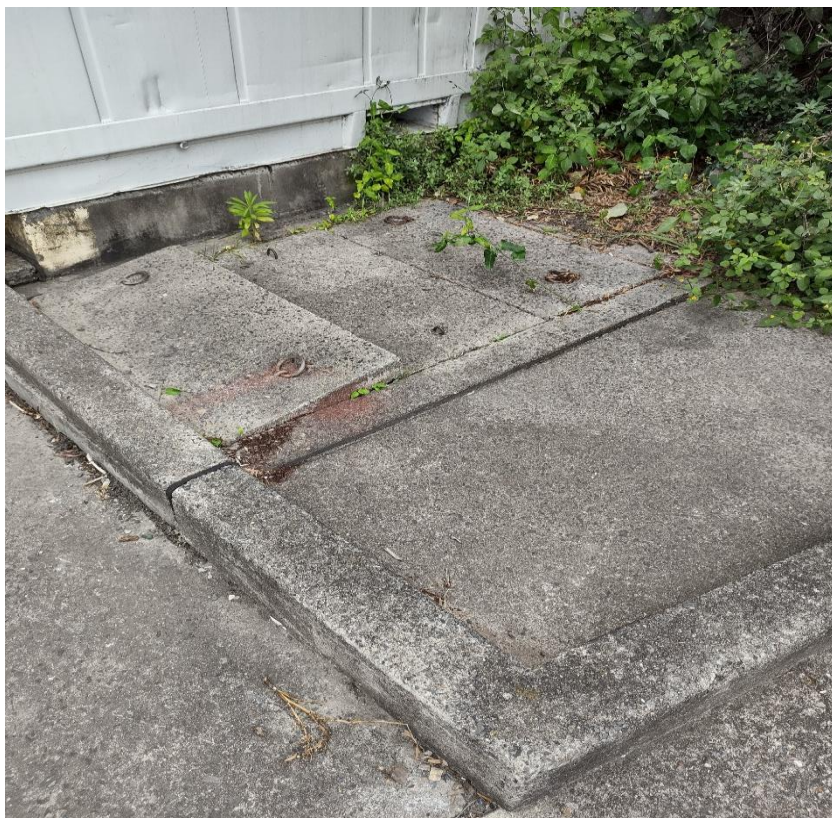
Photograph 2: Underground utilities access hatch
